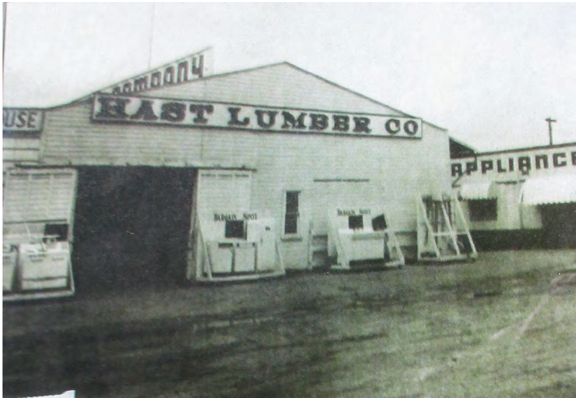
One of the original Hast Lumber buildings on the property that is no longer extant (Source: Commerce City Historical Society)
