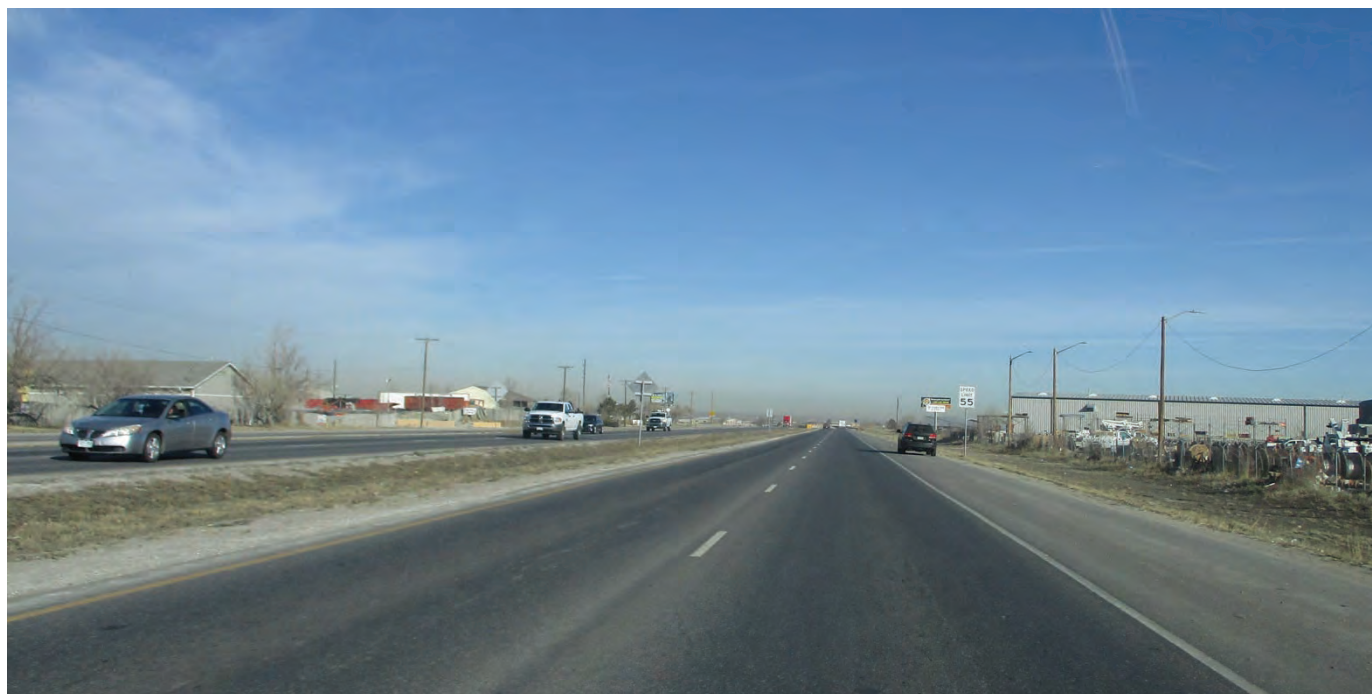
5AM3924.3_4: Looking north along US 6 north of the intersection with 77th Ave.
