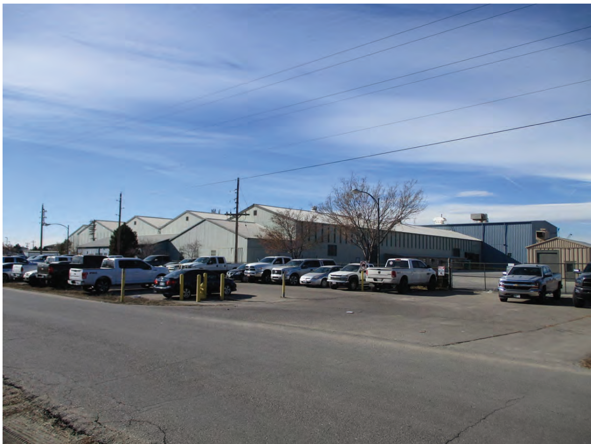
5AM4077_6.jpg: Looking southwest at 5AM.4077 main building from Dexter St. (January 24, 2020)
