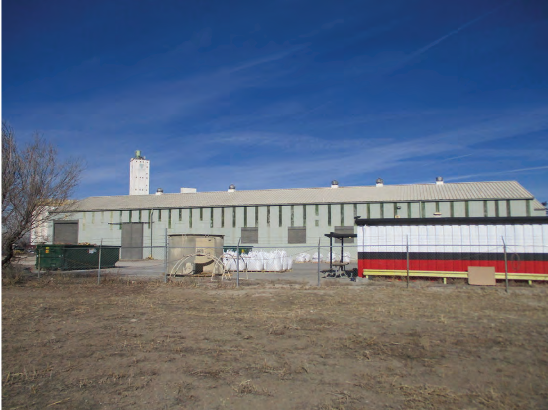
5AM4077_4.jpg: Looking north at 5AM.4077 main building and Building B from parking lot on adjacent site (January 24, 2020)
