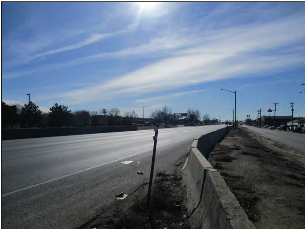
LOOKING SOUTH ALONG VASQUEZ BLVD. TOWARD PARKWAY DR./E. 60 TH AVE.
