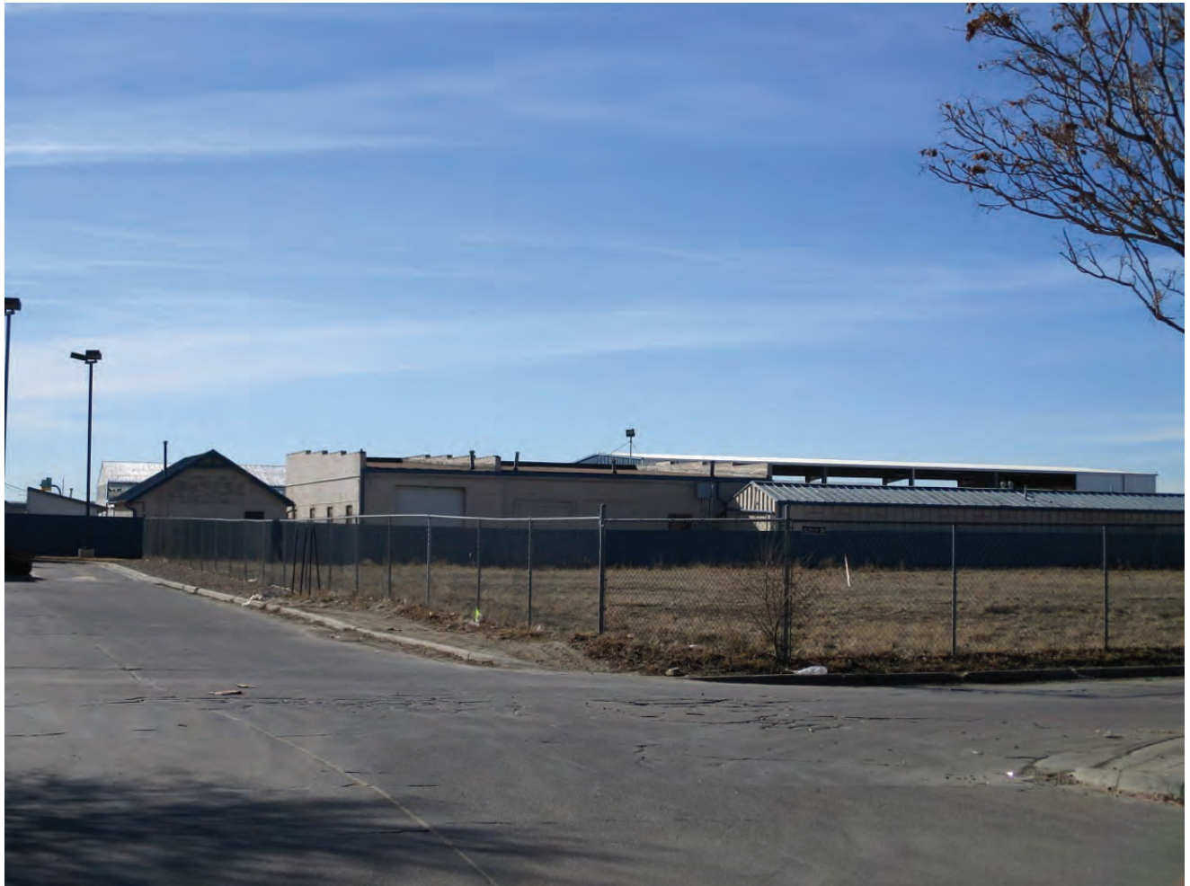
5AM4071_3.jpg: Looking south at 5AM.4071 from driveway on north adjacent site (January 24, 2020)
