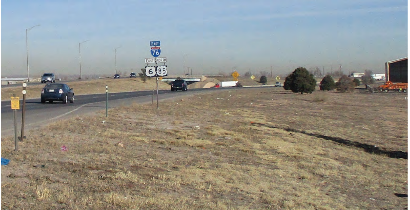
5AM3924.3_5: Looking north at US 6 near project's northern terminus at I-76 (January 24, 2020)
