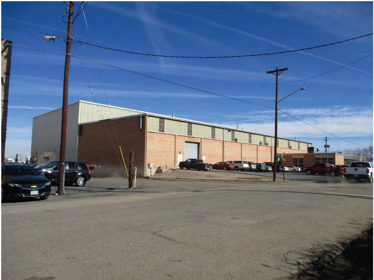
5AM4083_2.jpg: Looking northeast at 5AM.4083 from E. 63 rd Ave. (January 24, 2020)
