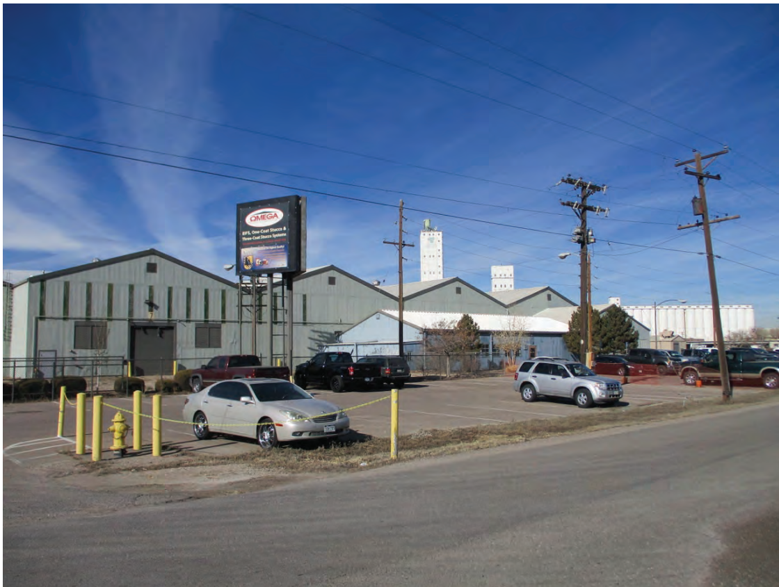
5AM4077_5.jpg: Looking northwest at 5AM.4077 main building from Dexter St. (January 24, 2020)
