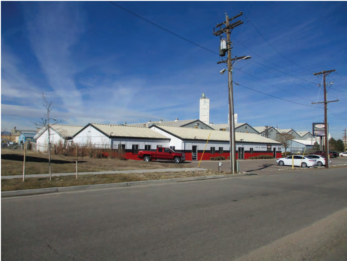
5AM4077_1.jpg: Looking northwest at 5AM.4077 Building A from Dexter St. (January 24, 2020)
