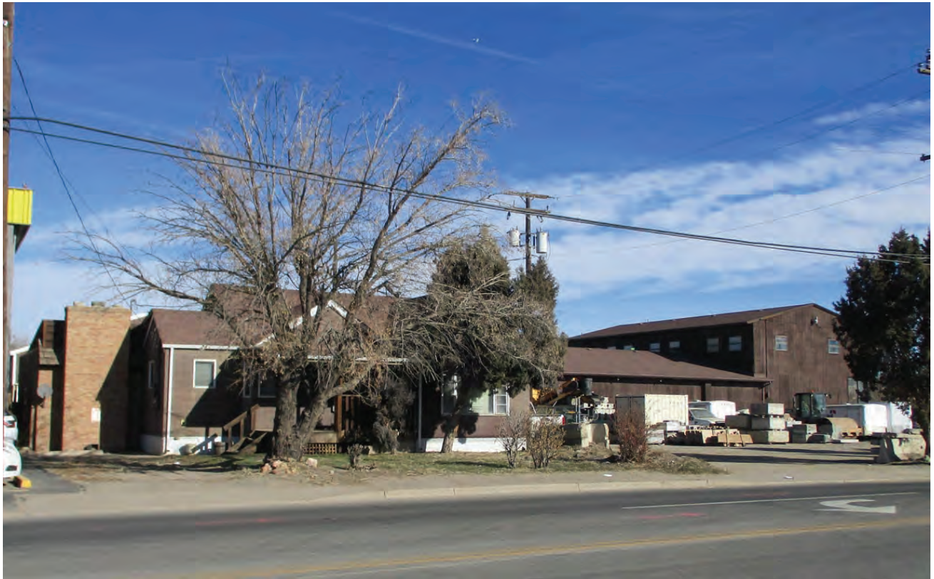
5AM4074_1.jpg: Looking northeast at 5AM.4074 from E. 60 th Ave. (January 24, 2020)
