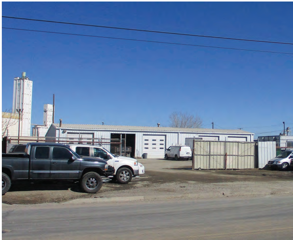
5AM4076_1.jpg: Looking north at 5AM.4076 from E. 60 th Ave. (March 3, 2021)
