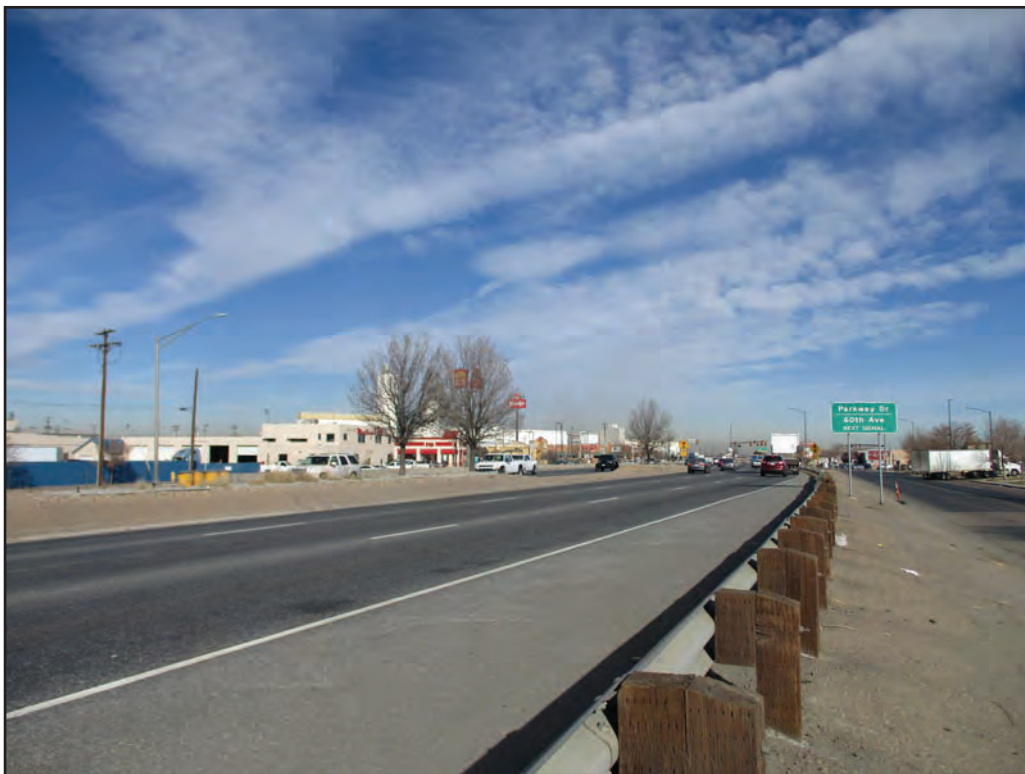
LOOKING NORTH ALONG VASQUEZ BLVD. TOWARD PARKWAY DR./E. 60 TH AVE.
